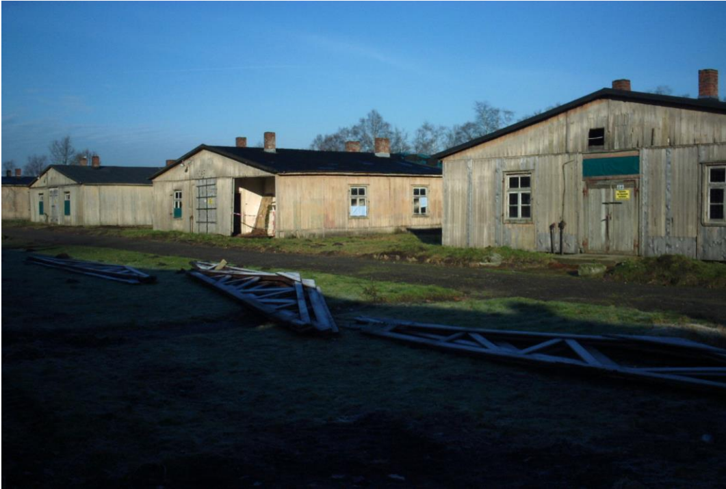
The facades of barrack Z4, Z5 and Z6
